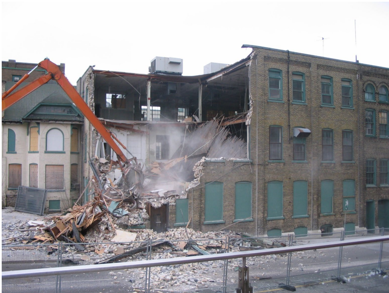
Demolition of the Forsyth Shirt Factory, Kitchener
